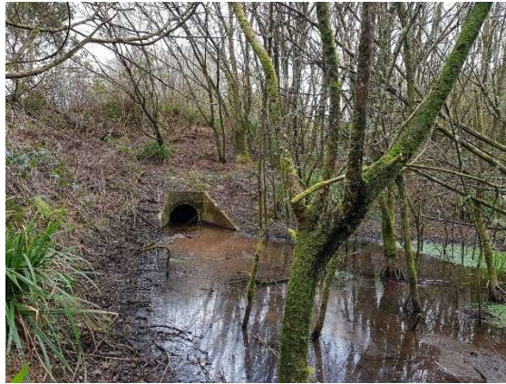
Figure 2.5: Upstream inlet to culvert from wet woodland area.
