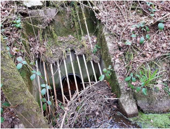
Figure 2.4: Upstream inlet to culvert from northern attenuation pond.
