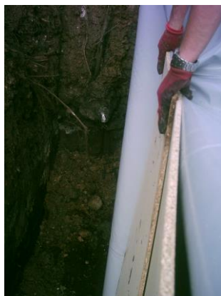
Figure 4 Construction of the Japanese Knotweed containment area
