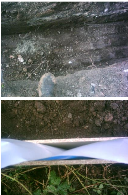
Figure 4 Construction of the Japanese Knotweed containment area
