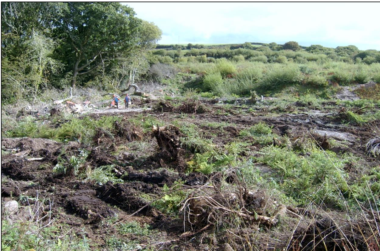
Figure 2 The cleared southern end of the site - May 2011
